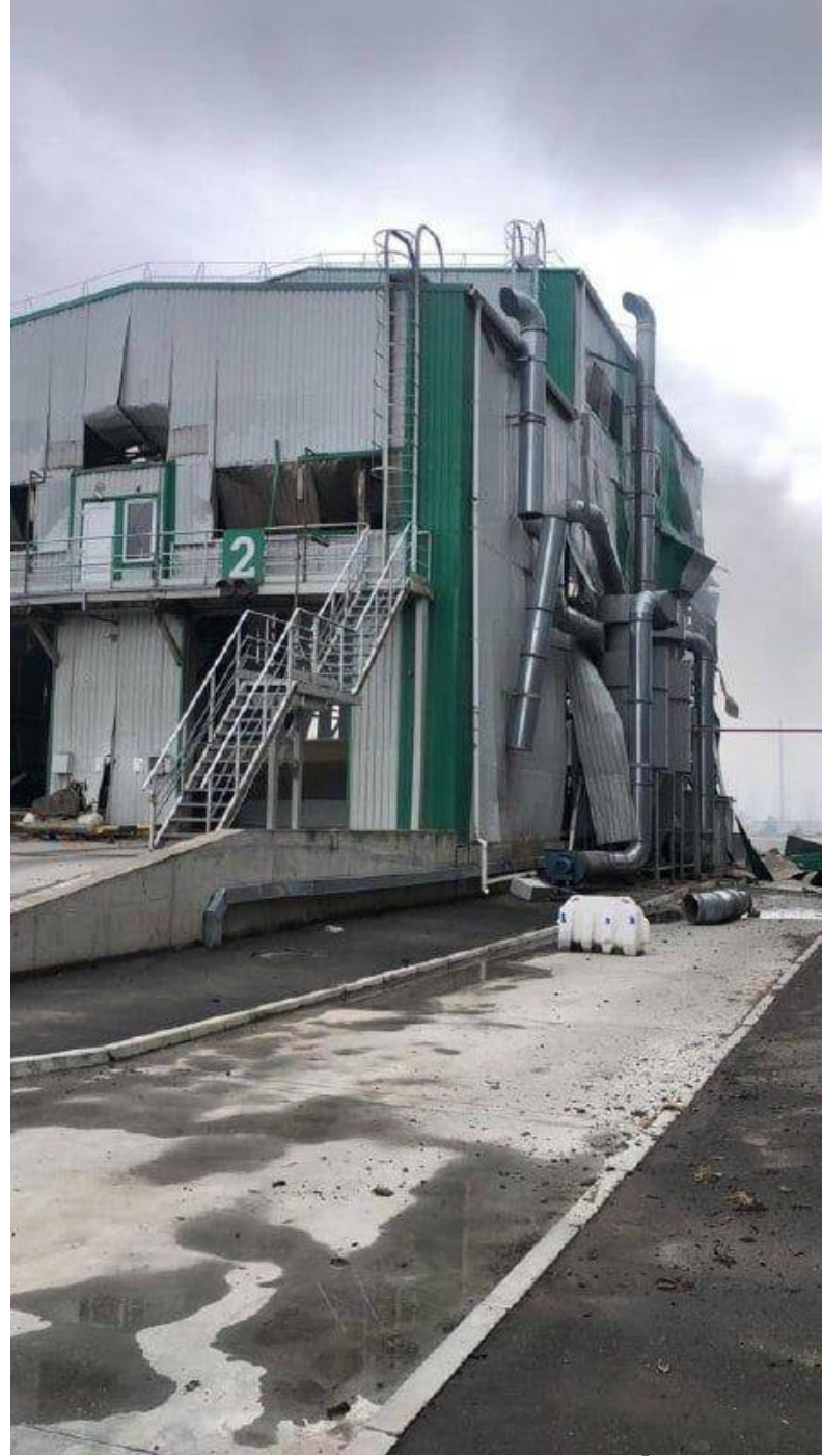
PAEK silo, Mykolaiv region
